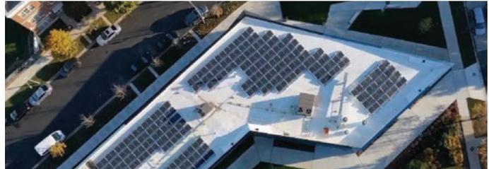
*Through a generous donation, the Center has solar panels secured to roof that will generate 58% of its power needs.*
